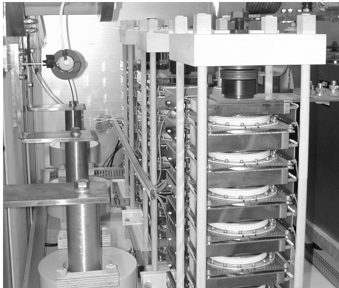
Figure 2: Arrangement of semi-conductor switches in the pulsed current plant
