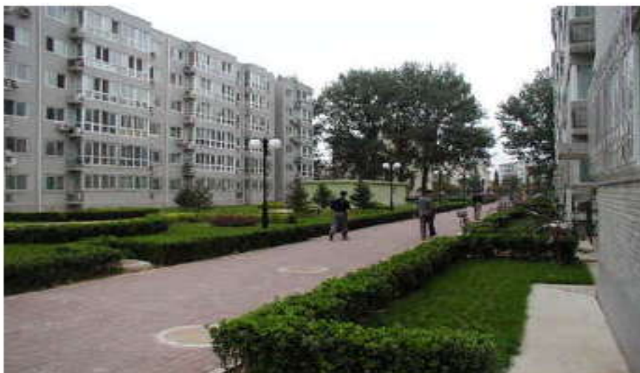
Figure 7-1 Appearance of Tianxiu Garden
