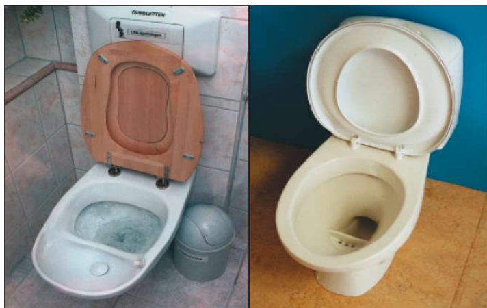
Figure 5-7 Separating-toilet installed in Understenshjäden and Palsternackan of Sweden (Johansson, 2001)
