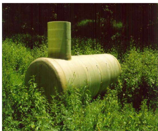
Figure 5-9 Holding tank (left) (Johansson, 2001)
