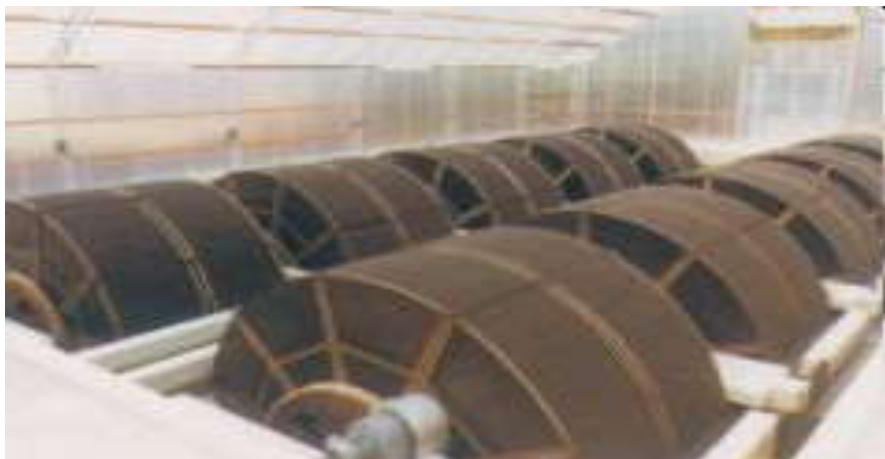
Figure 4-4 Schematic of RBC (Huber, 2002)
