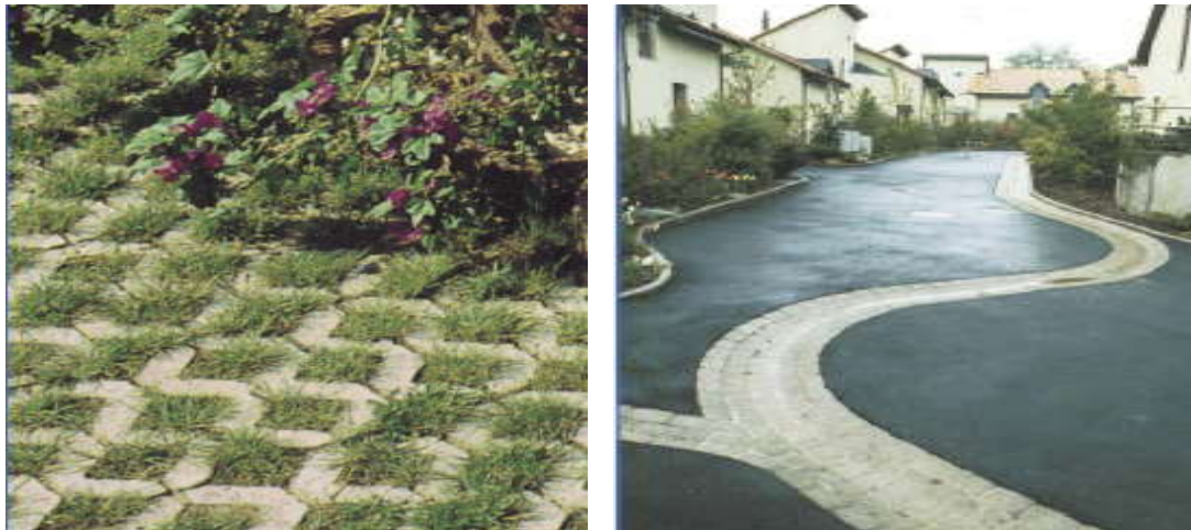
Figure 6-5 The green land with grass for rainwater infiltration (left) and permeable surface for rainwater infiltration (right) (Broschüre Stadt Landshut, 2006)
