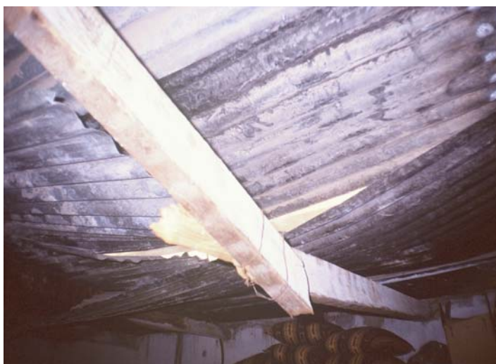
Figure 3.3: Image of Gaza camp in Jordan / cramped building structures
