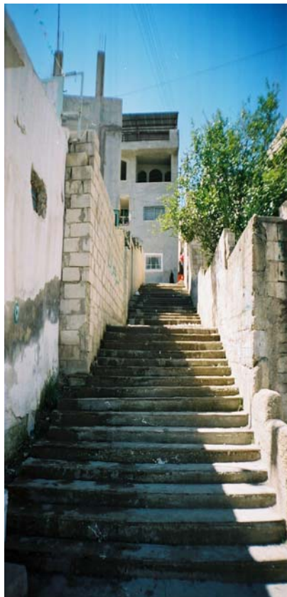
Figure 3.6: Renovation of stairs pedestrian paths as type of upgrading process
