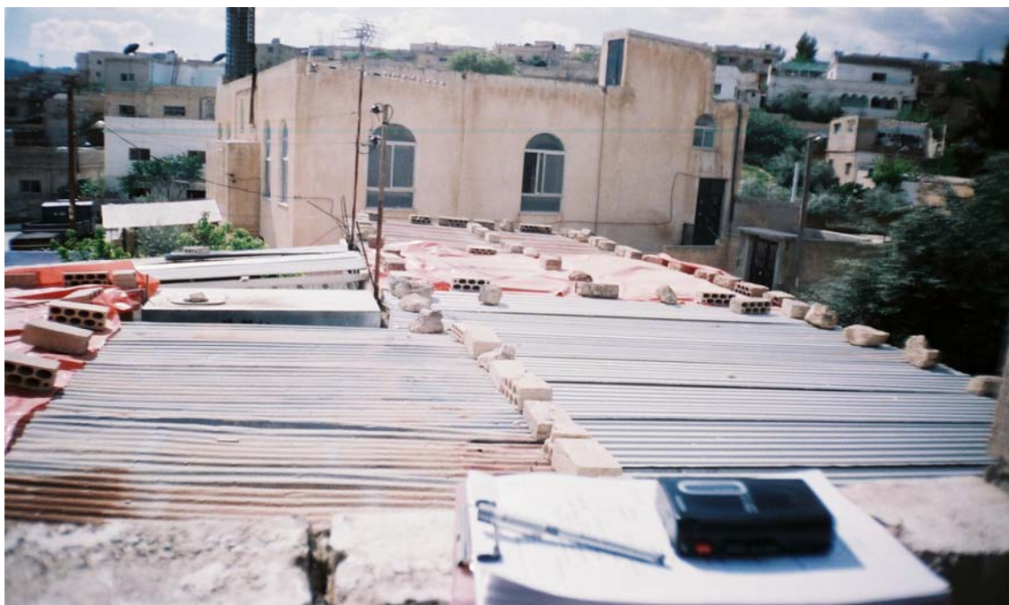
Figure 4.6: Upgrading in Suf camp – still deteriorated conditions
