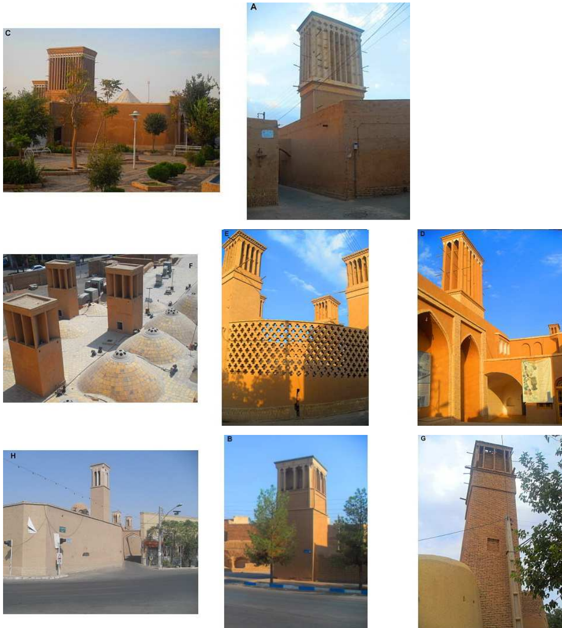
Fig. 5-13: Different types of Badgirs in the central cities of the Iranian Plateau: A, C, D, and E are some of the Badgirs of Fahadan neighborhood in Yazd. G is a renovated one in Naein. F shows the Badgirs of Amir-Chakhmagh Mosque in Yazd. Source: author.
