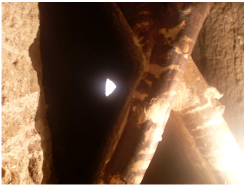
Fig. 5-16: X-shaped inner blades of the Badgir of Tabatabaee House in Kashan. The photo is taken from down to top of the inner space of Badgir. Source: author.
