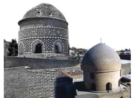
Figure 3-37 Kheshty Dome, before and after renovation Ref: Rezvani; In search of urban identity: Mashad, 1384 AHS/2005 AD
