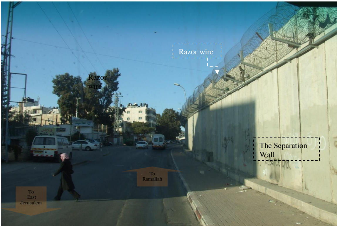
Figure 5.36: Poor structure of the major road used by Palestinians to enter East Jerusalem from West Bank, (researcher)
