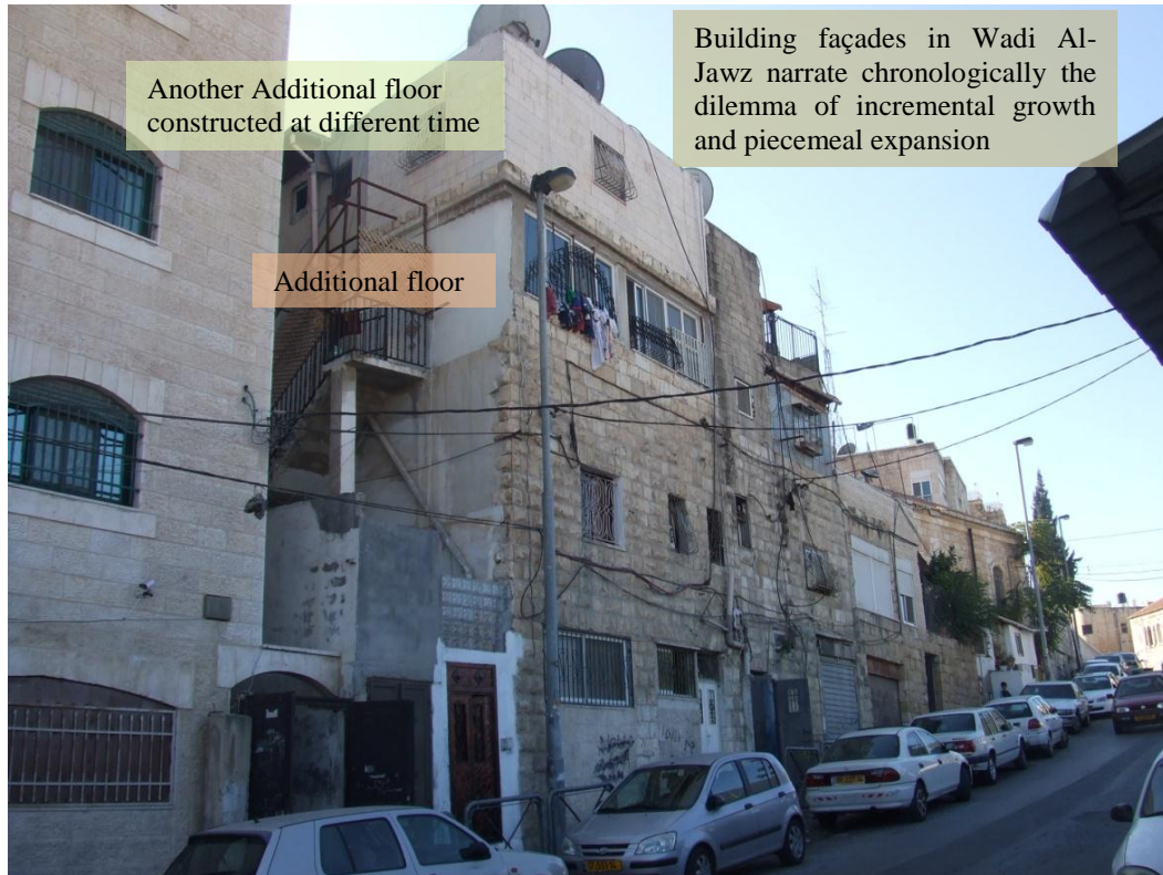
Figure5.65: Heterogeneous building façades in Wadi Al-Jawz – an output of the political architecture, (researcher)
