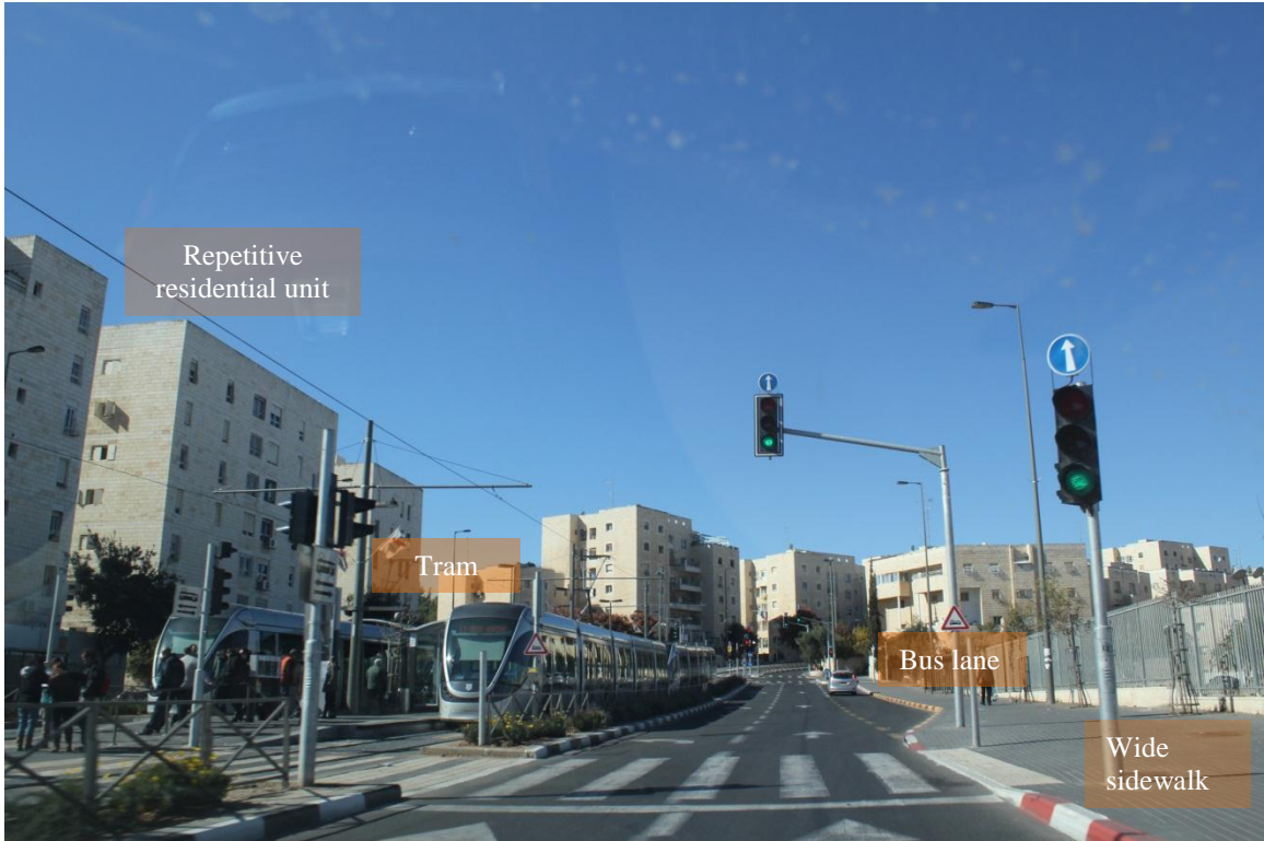
Figure 5.30: High-tech infrastructure in Pizgat Ze'ev Jewish settlement in East Jerusalem, (researcher)
