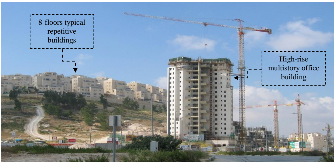
Figure 5.50: High rise tower under construction in Har Homa settlement, (Halawani, 2006, edited)
