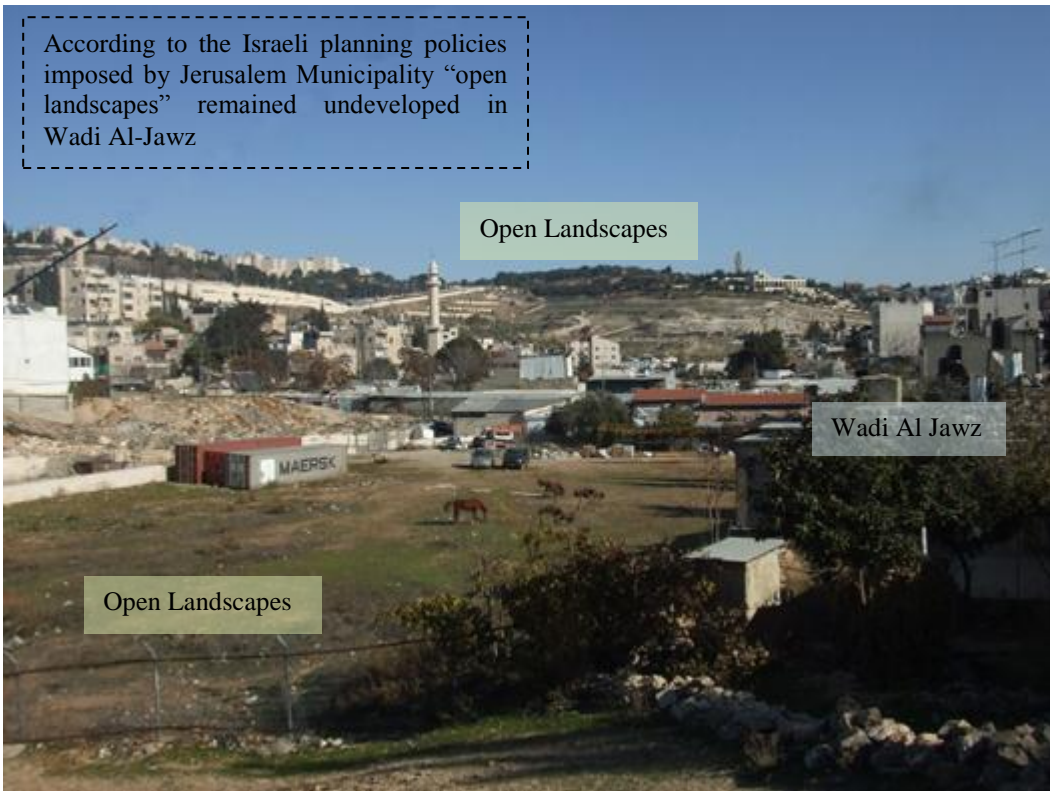
Figure 5.73: Open landscapes in Wadi Al-Jawz remained undeveloped despite the vital need for expansion, (researcher)
