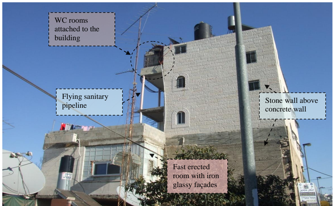
Figure 5.64: Incremental growth, sanitary rest rooms attached into residential building in Wadi Al-Jawz, (researcher)
