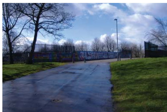
Plate 19 - Graffiti art on guard wall of the bridge over the railway. View towards south of Ward End Park. Photo by NK 2010.
