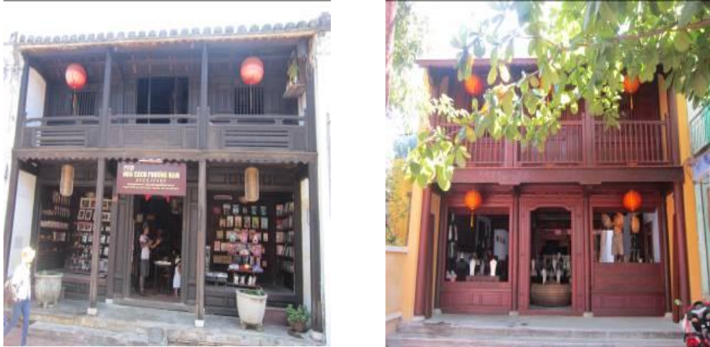
Photo 3.4: Wooden Old House in Quang Nam Province
