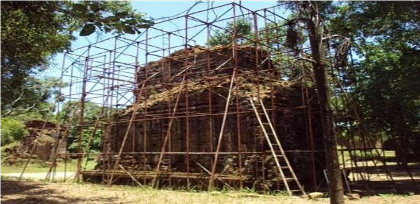
Photo 7.5: A Broken My Son Tower after Big Flood in October 2011
