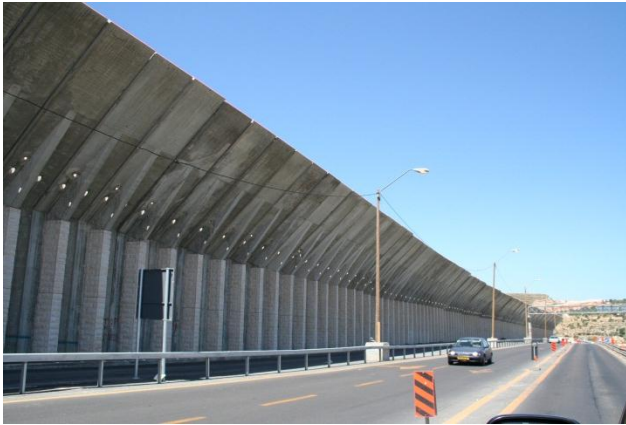
Figure (2.7): Section of the Segregation Wall West of Bethlehem City-area along Bypass Road no. 60
