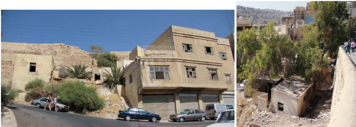
Deteriorated buildings on the Citadel slopes
