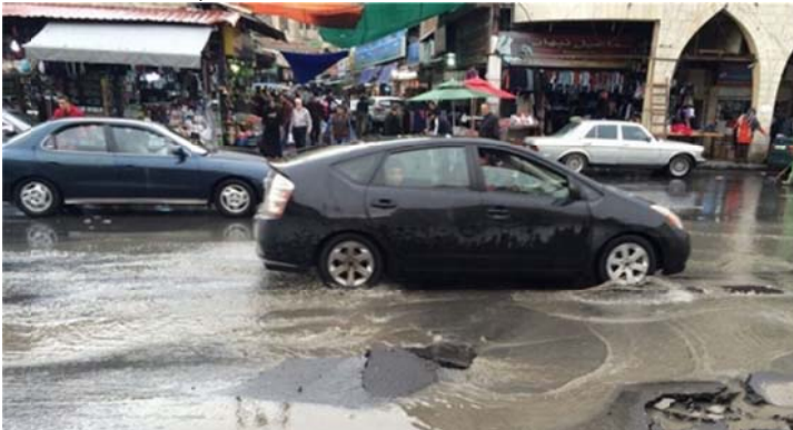
Storm water flooding in the Downtown , Jafra News (2015)
