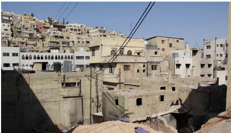
Deteriorated buildings at the Downtown
