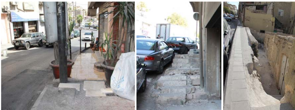
Figure 60: bad conditions of sidewalks
