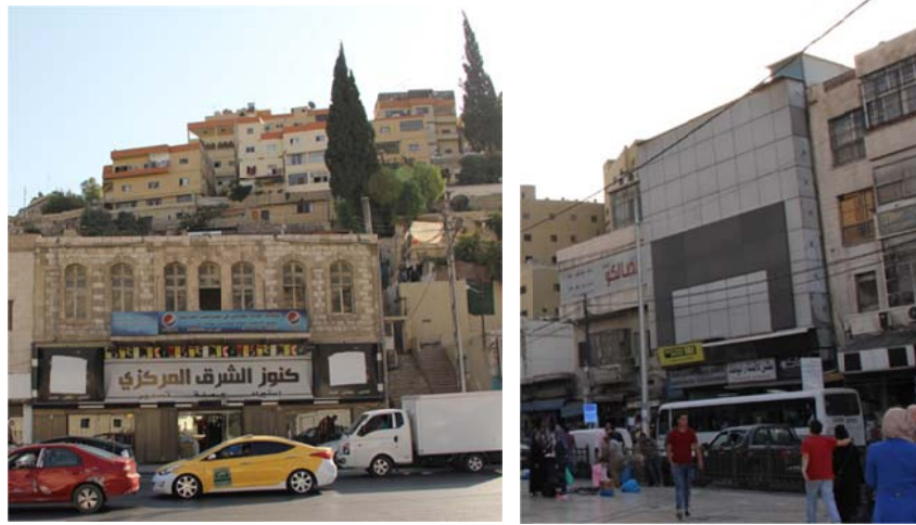
Photos show inappropriate signage and building materials
