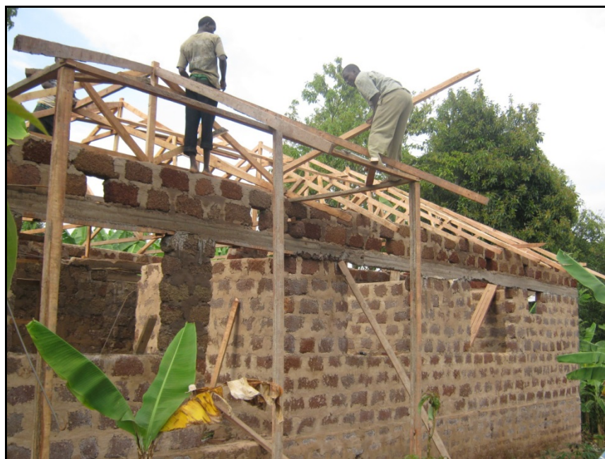
Figure 8.2: Timber used as the roofing (rafter) materials in Moshi district.
