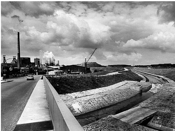
Figure4. 7 Emscher River,1960 as an open wastewater through a densely populated industrial region. Source: http://www.eglv.de/en/water-portal/home/
