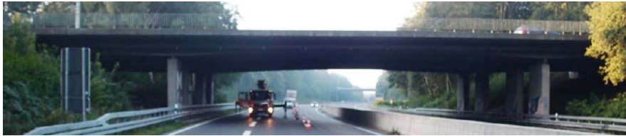
Fig. 2: Bridge view during the installation of the monitoring.
