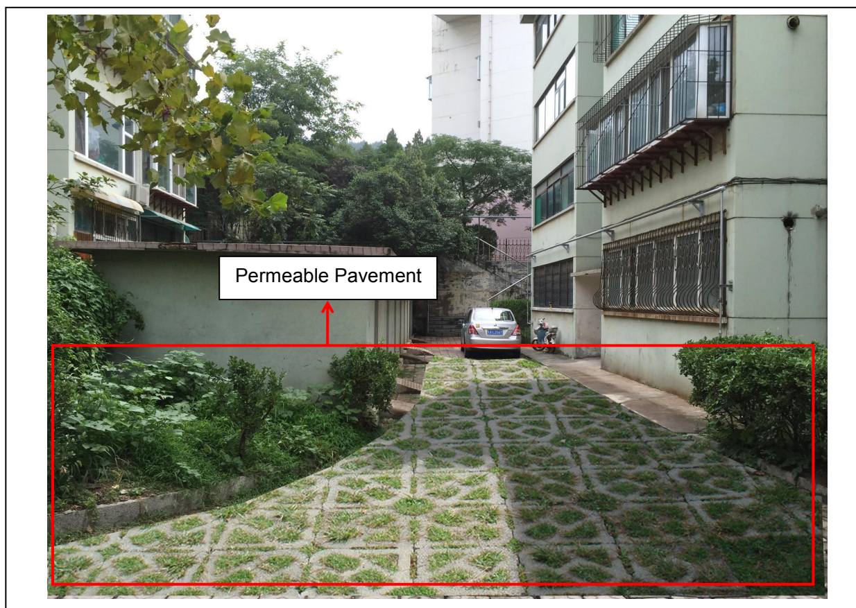
Figure 4-14: Permeable Pavement replacing the damaged road pavement (Source: WRISD, China)
