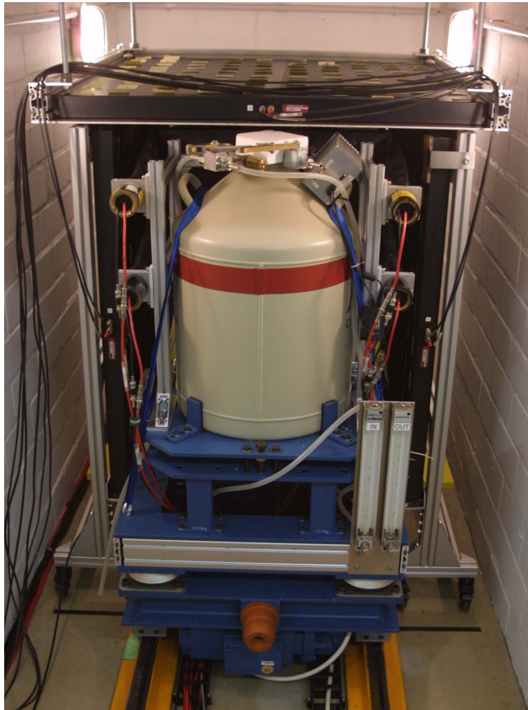
Figure 6.12.: The inner shielding of the DLB at the measuring position underneath the cast iron ceiling. The completely upgraded muon veto detector is installed. Black scintillation detectors are mounted in aluminium support structures. The blue wagon can move the inner shielding alongside the orange rails on the floor. In the foreground is the grey liquid nitrogen reservoir, the yellow inner shielding is not visible due to the coverage of the muon veto.
