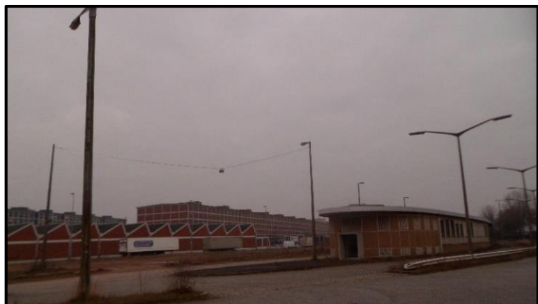
Figure 17 Vacant Industrial Buildings in Bremen (Original)
