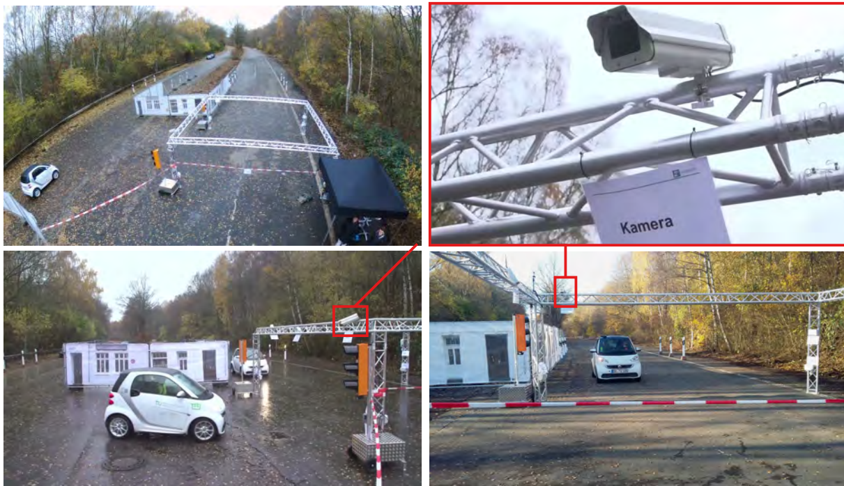
Figure 3.3: Overview of the InVerSiV field test with the road side unit camera platform. The cameras monitor the traffic scene from a stationary truss structure.
