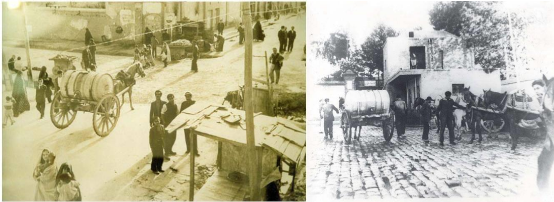
Figure 112 Supplying water using water tanks (Najafzadeh, 2021)
