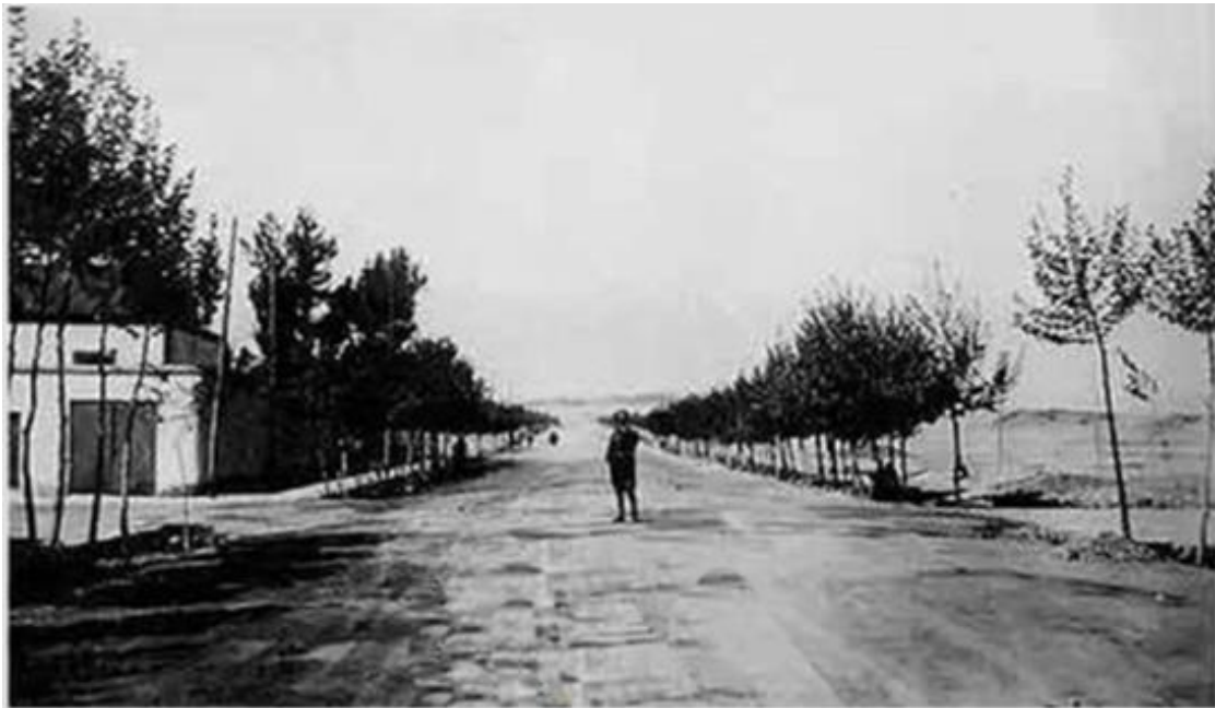
Figure 126 Constructing new roads in the city of Tehran by Reza Shah in 1946 (Mohammad Reza Pourzargar, Parichehr Moafi Ghaffari, Maryam Amjadi, 2018)
