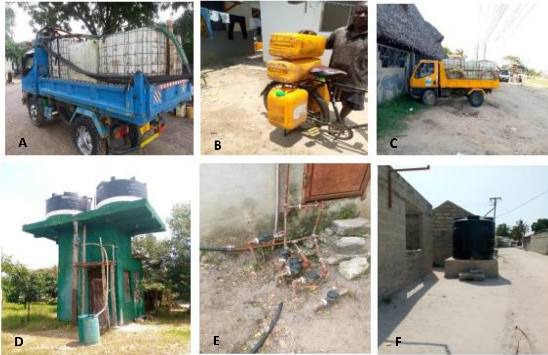
Figure 5.1 Non-utility-networked water infrastructures; (a) non-registered private tanker trucks, (b) Bicycle utility water reseller, (c) Utility registered tanker, (d) Privately mechanized boreholes for in-house/pipe water connections, (e) pipelines and meters of private boreholes networked, (f) standalone reseller of utility's water to neighbours.
