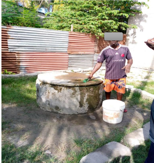
Figure 3.4 Protected bore well
