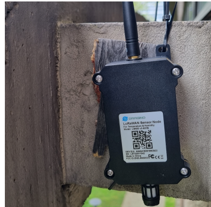
Sensor 4 at the library's south facade
