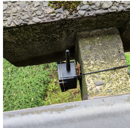
Sensor 2 at the library's north facade
