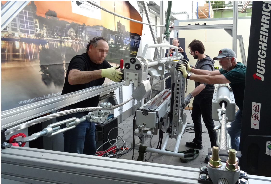
Figure 6.5: Installation of DSRs in the scaffold
