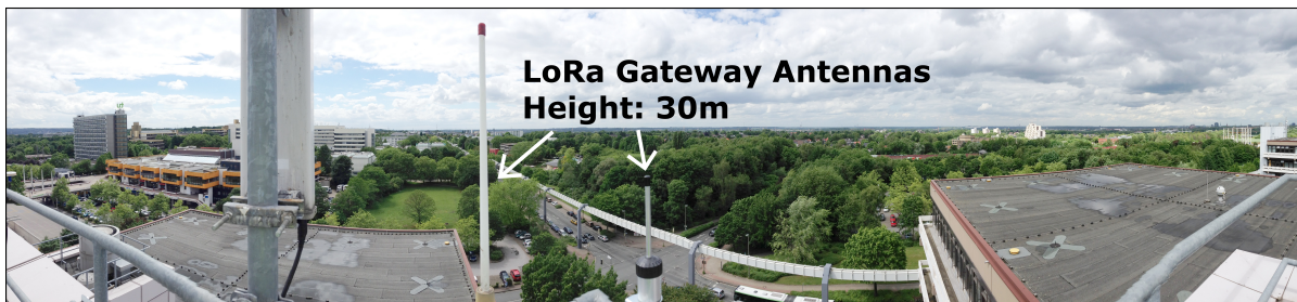
Figure 1: Installation site of Smart City LoRa Gateway antennas in 30 m height.
