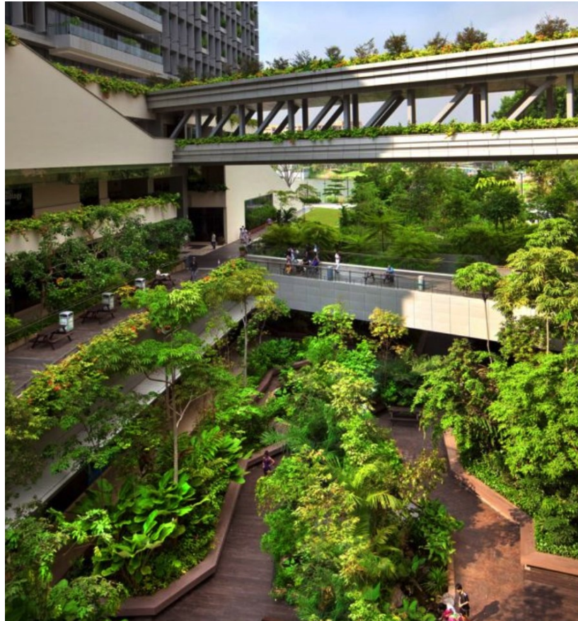
Image 15 – Khoo Teck Puat Hospital, http://www.greenroofs.com/projects/khoo-teck-puat-hospital-ktp/h/
