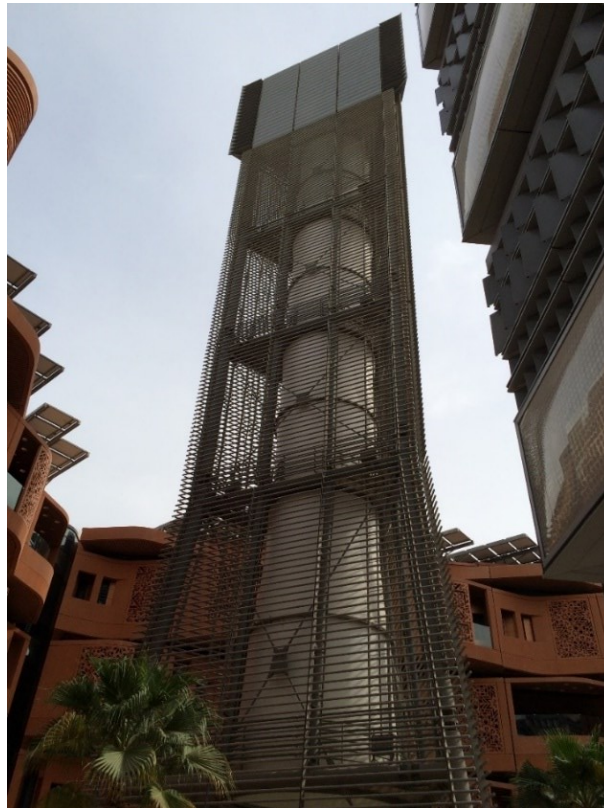
Image 10 – Masdar City – Wind tower for cooling, author's study trip to Masdar in 2015
