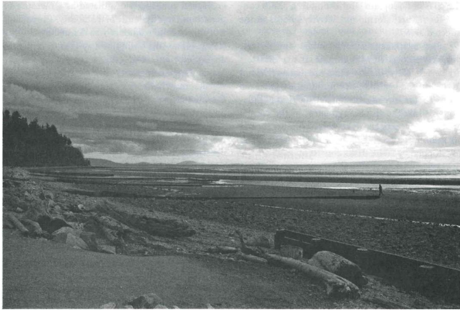
Figure 22.4 This older breakwater infrastructure at Crescent Beach, Surrey, will not be sufficient to hold back the rising sea level of the next 20 years. This realization prompted Surrey to undertake the Coastal Flood Adaptation Strategy (CFAS).
