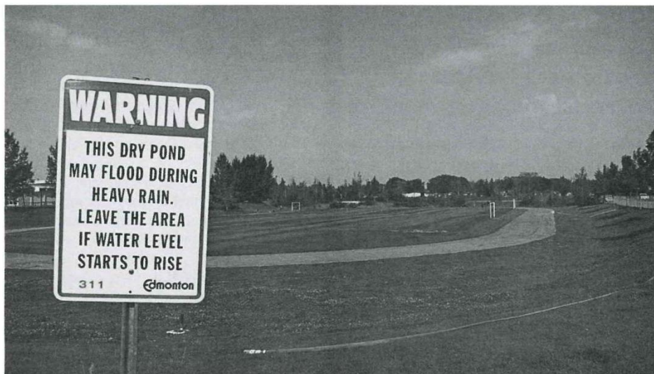
Figure 22.3 An example of climate adaptation infrastructure, this dry pond in a park in Edmonton is designed to also serve a stormwater management function.
