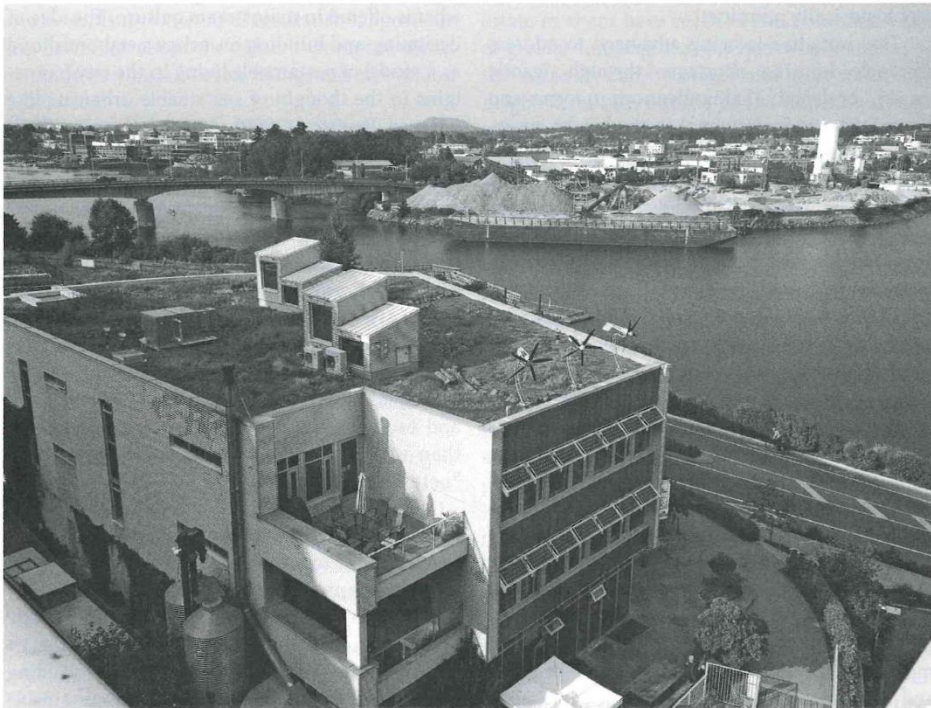
Figure 22.2 This building is a cornerstone of the Docksider Green model sustainable neighbourhood in Victoria, BC. In addition to its green building features, such as its green roof and solar and wind infrastructure, it also offers social features, such as the neighbourhood café and neighbourhood greenspace, as well as access to the Galloping Goose bike trail.
