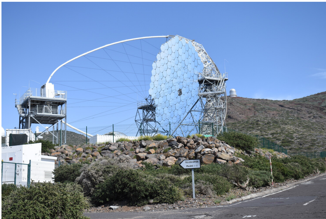
Figure 1.14: Photo of the LST-1 in the parking position during daytime in 2022. The camera is resting on the camera tower (left) and the mirrors are defocused.
