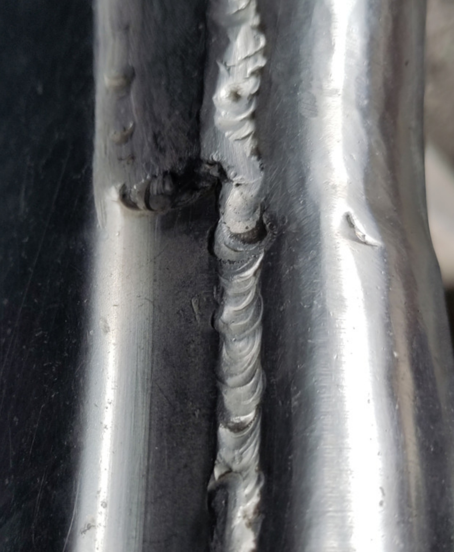
Figure 1.17: Welding seam — Welding creates a joining area of contact that contains the fusion line itself (where the material is melted) but also a heat-affected zone (where the material does not melt). Alteration of the latter microstructure can cause risks in the form of reduced tensile strengths. [129]
