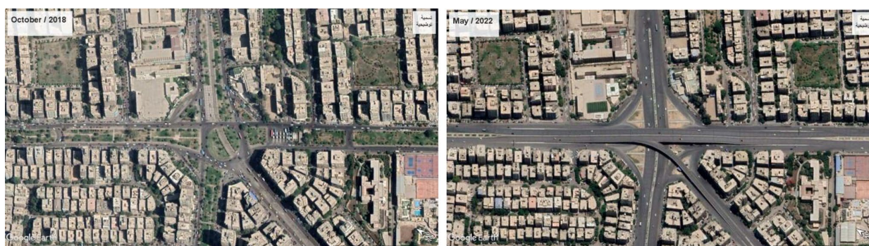
Fig. 1 Al-Hegaz Square before and after renovation. Both maps were exported from “Google Earth Pro”. The image on the left was exported in October 2018 and the one on the right in May 2022. no editing applied, and the difference between the colors of both satellite images is due to the conditions of each photo in Google Earth
