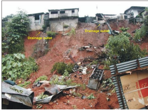
Picture 5. Sample photo of improperly built houses in Baguio City
