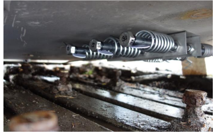
Figure 6 Coils installed underneath a cover plate. Source: IKS Dresden GmbH
