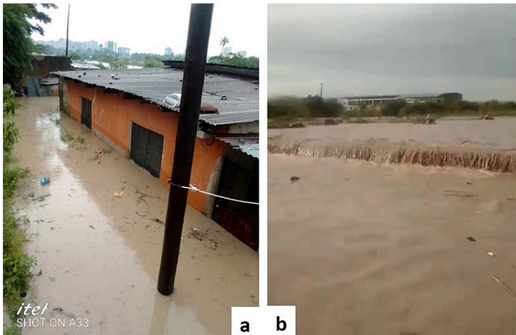
Fig. 15. Hananasif neighborhood along Msimbazi River (a); overflowed Jangwani Bridge on Morogoro Road and adjacent DBRT Depot (b).
