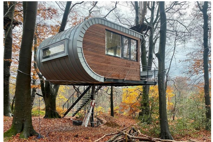
Figure 10 Foundation of a permanent building using inclined cables fixed on trees. Source: Ingo Muench/TU-Dortmund
