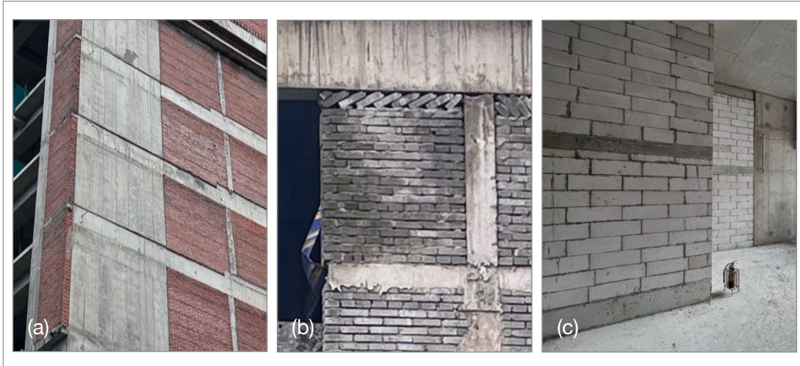
Figure 4.6: (a) Concrete-Brick Wall, (b) Wall-Slab/Beam Transition, (c) AAC Walls
