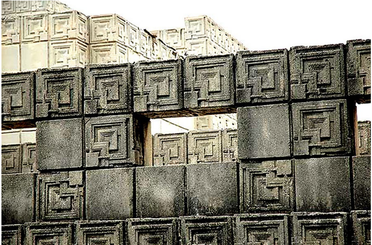
Abb. 19: Frank Lloyd Wright, Ennis House, textile blocks, Los Angeles, 1924 © Alan M. Pavlik
