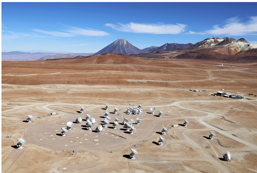
Figure 2.3: An overview of the Chajnantor Plateau in the Atacama desert in Chile. Several of the 66 antennas and 192 antenna foundations can be seen. The antennas can be repositioned to vary the interferometer layout and baseline lengths. [24]
