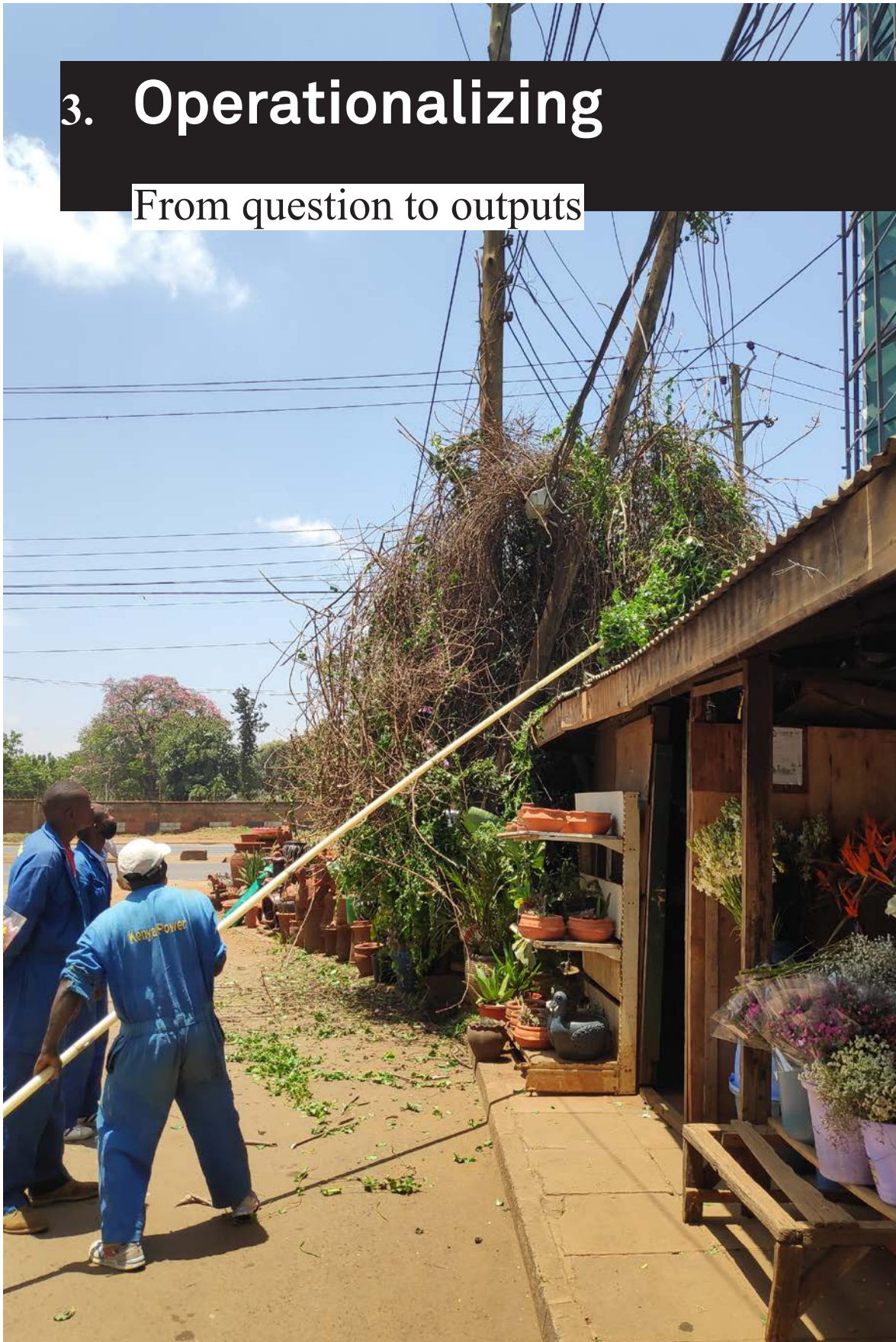
Figure 8: KPLC workers remove overgrowth from power lines; photo by author (2022).
