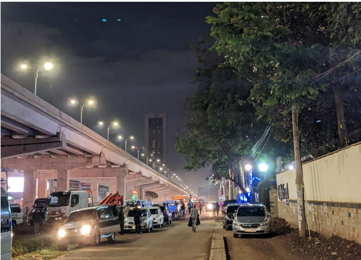
Figure 3: Nairobi Expressway at night in Westlands; photo by author (2023).
