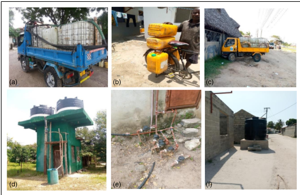
Figure 1. Water supply infrastructures beyond the utility network; (a) non-registered private tanker trucks, (b) bicycle utility water reseller, (c) utility registered tanker, (d) privately mechanized boreholes for in-house/pipe water connections, (e) pipelines and meters of private boreholes networked, (f) standalone reseller of utility's water to neighbours.
