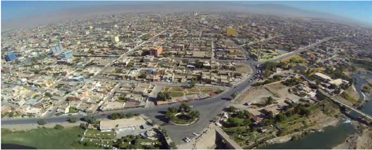
Figure 11- 51: Aerial Photo of Zakho Source: University guide of Zakho, 2015, P. 5.
