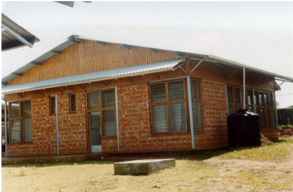
Appendix 4: Perspective showing the west and south side of the administration building (refer to figure 3.1)
