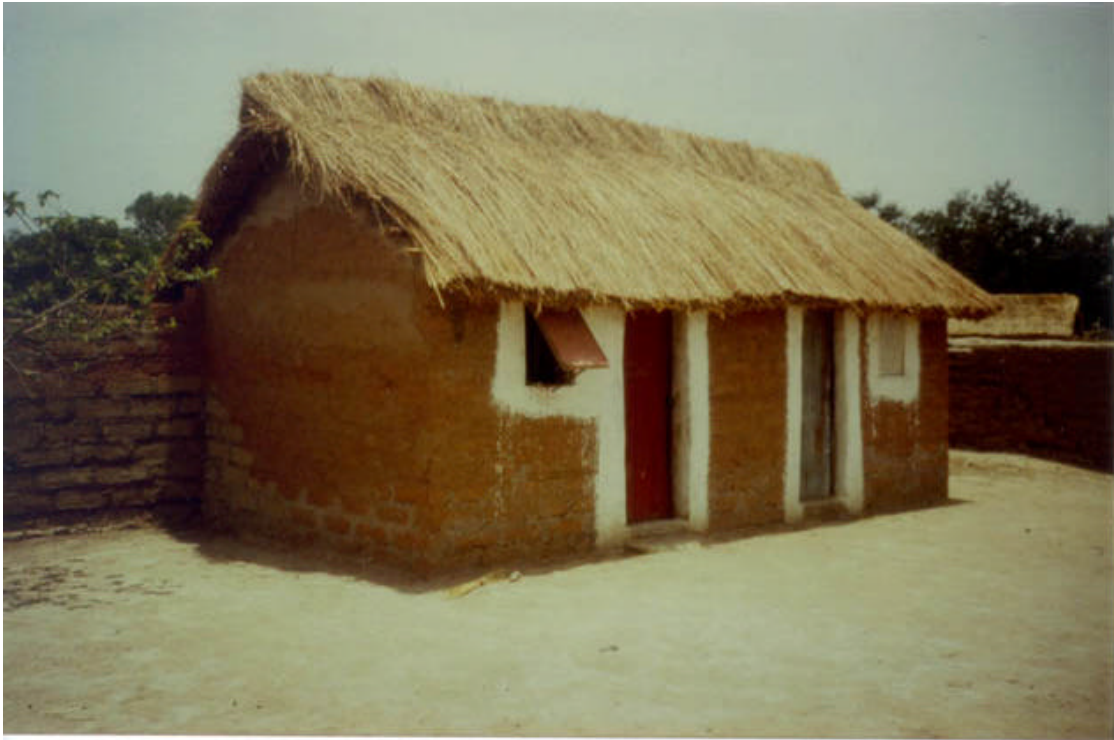
Figure 4.9: Dwelling building with wooden (opaque) windows in hot and humid tropical regions
