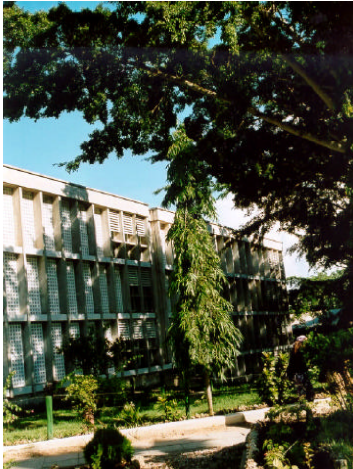
Figure 6.15: Trees providing additional shade to the administration building at the University of Dar es salaam
