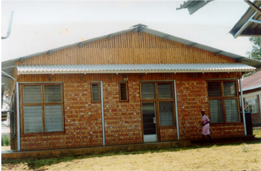
Appendix 5: Elevation of the west side of the administration building (refer to figure 3.1)
