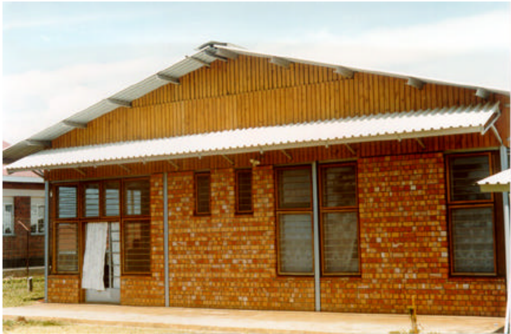
Appendix 3: Elevation of the east side of the administration building (refer to figure 3.1)
