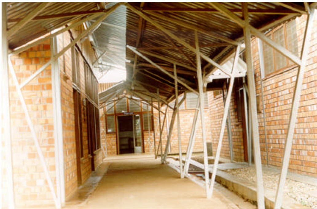
Appendix 2: View of the roofed walk way connecting different buildings of the private wing
