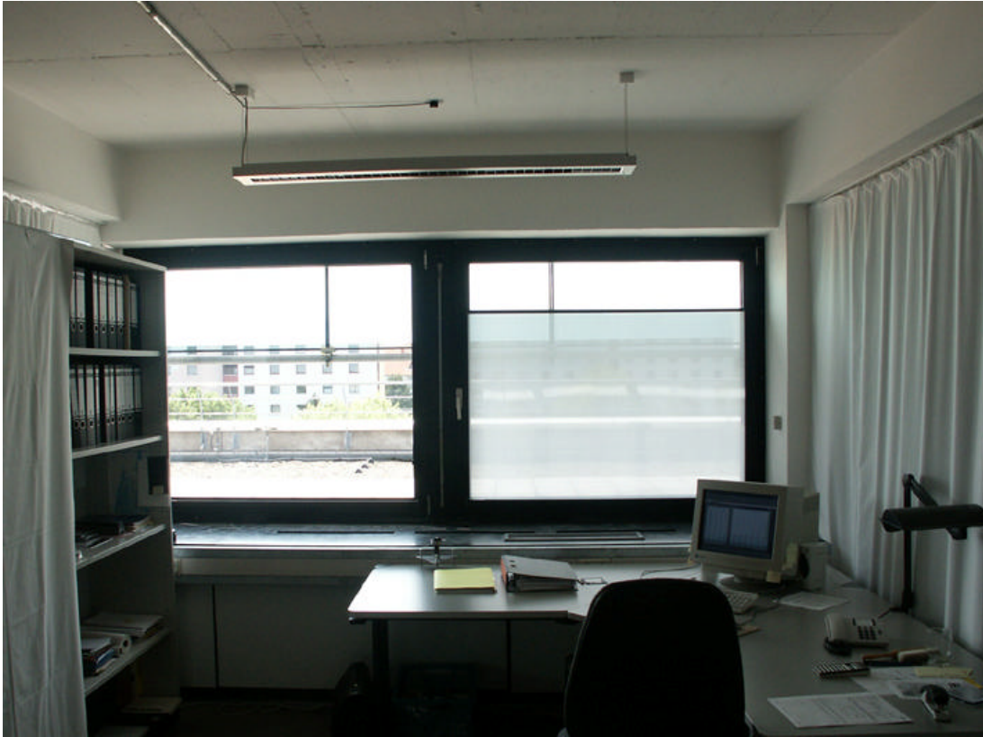
Figure 5.6: Transparent glare screening device installed on the inner side of the window
