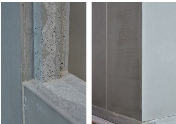
Fig. 18 Physical prototype of the one-to-one demonstrator showing the water-repellent surface and joining quality
