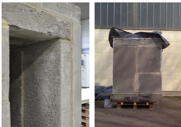
Fig. 16 Long-term monitoring of the demonstrator to prove the performance of the building physics, building structure and joining techniques
