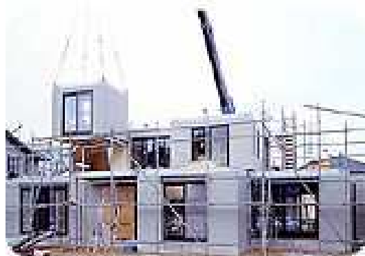
f – installation of units at site
