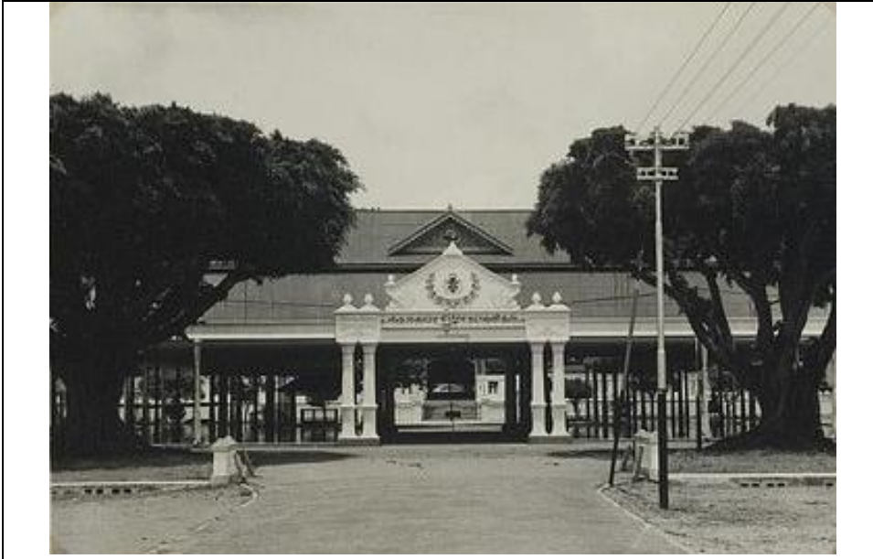
Figure 5-10. Pagelaran hall of kraton Yogyakarta in 1939 - A mixture of steel-concrete construction and traditional ornamentation
