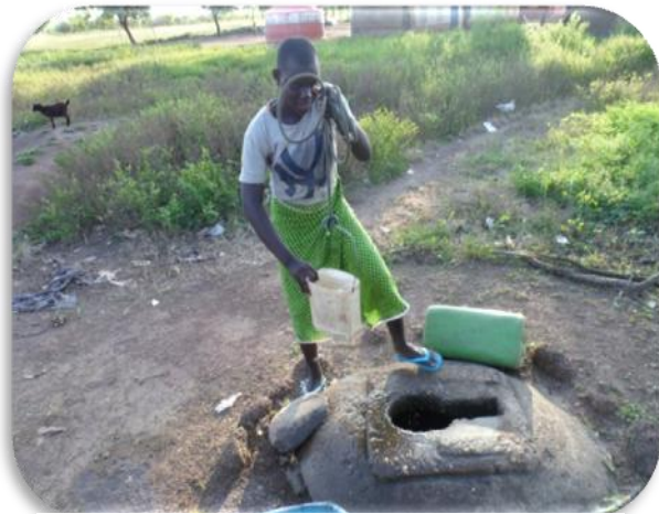
Figure 7.10: Pit Latrine Used as a Well
