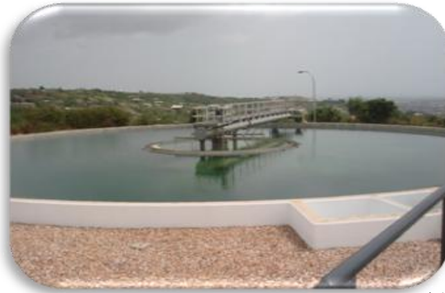
Figure 3.14: Water Treatment Plant at Dalum, Northern Region
