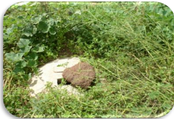
Figure 7.13: Abandoned Sanitary Facility in Damdo
