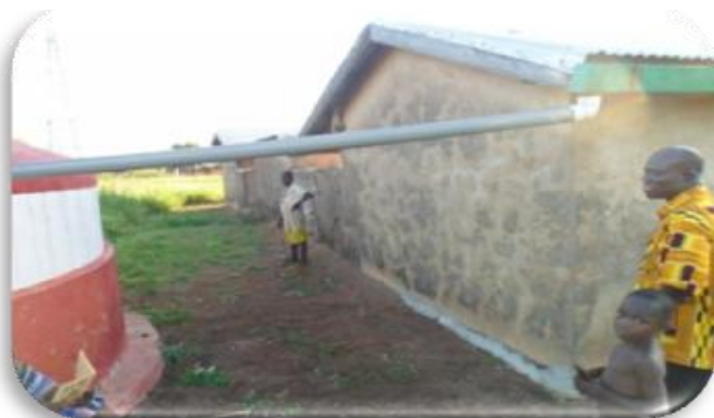
Figure 7.6: A Rain Harvesting Tank for a Teacher's Quarters in Wambong, Yendi Municipality
