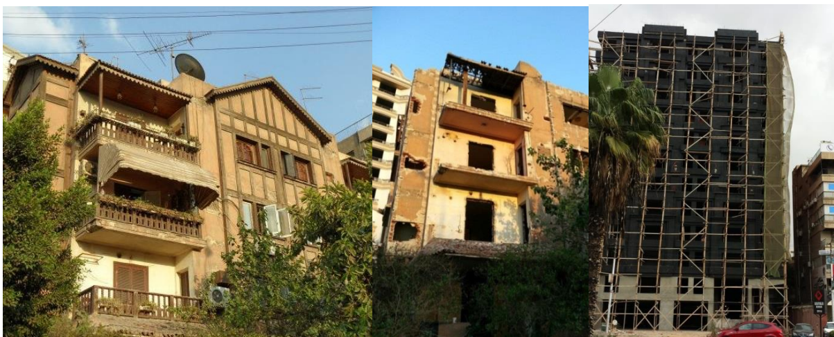
Figure 11-14 Swiss Chalet: Left: showing the unique architectural style of the building (Michel Hanna, 2012) Middle: Vandalism expropriating the building form its ornaments intending demolition, (Michel Hanna, April 2013) Right: High-rise under construction replacin
