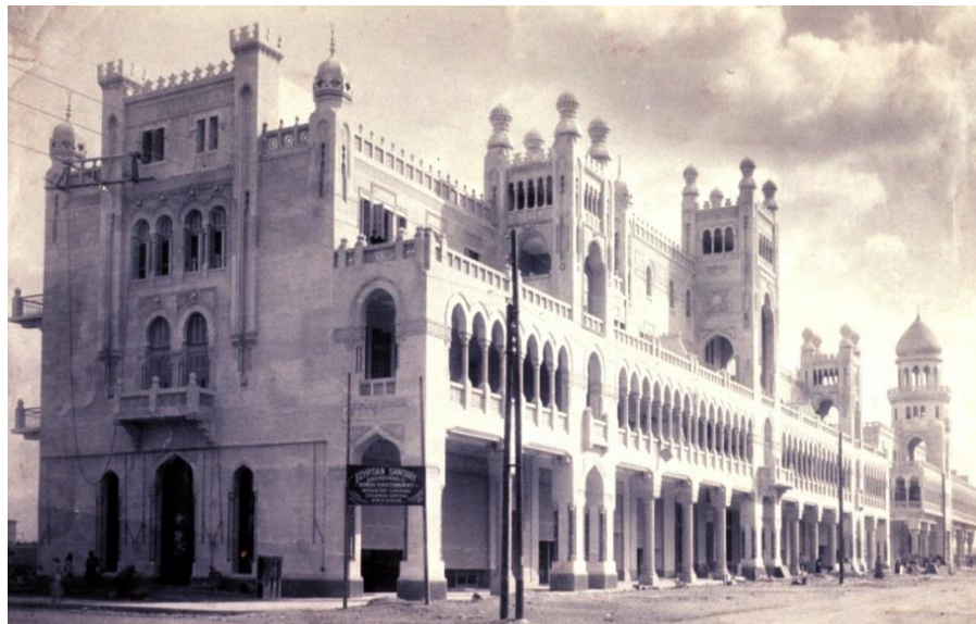
Figure 3-13 Heliopolis Oasis Company Ibrahim Laqani Street, Arcade Building with Neo-Islamic and Moorish style, designed by Ernest Jasper 1908-09 , Source: AN/IFA Paris (GOPP-URBAMA Report, 2000)
