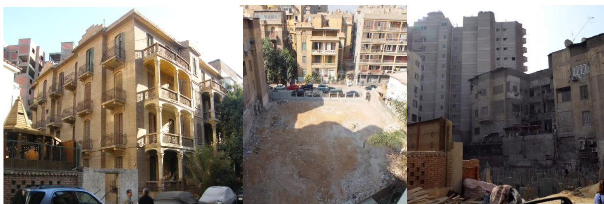
Figure 11-8 Left: Registered building, 3 Maspeero St., Heliopolis (NOUH, 2010) Middle: empty Plot after building torn down (NOUH, 2012) Right: Construction of a new building instead (Michel Hanna, October, 2014)
