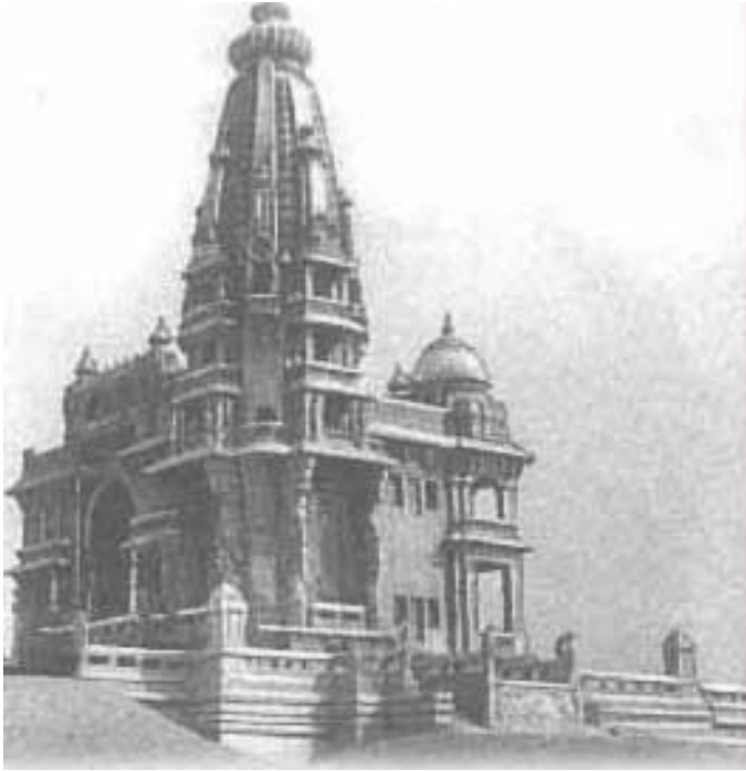
Figure 3-4 Baron Empain Palace Designed by Alexander Marcel 1907-11 source: http://www.egy.com/community/95-05-13.php
