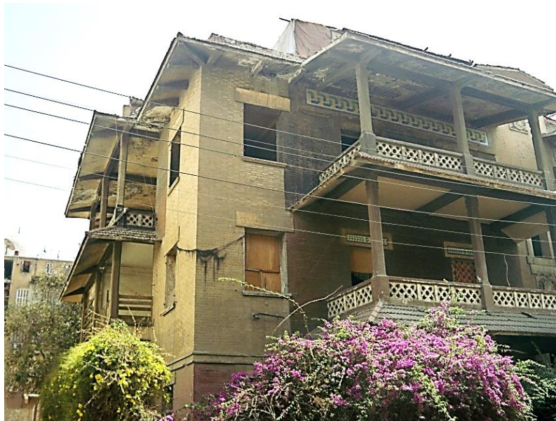
Figure 1-7 3 Soumal Street, Heliopolis deliberately deserted villa waiting for an opportunity to tear it down. Photo by author, 2013
