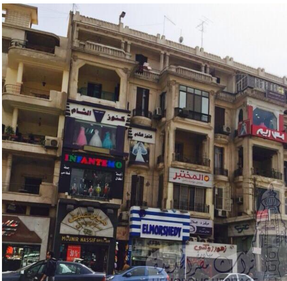
Figure 11-10 Store Elevations in a distinctive building in Heliopolis photo: HHI, March 2015
