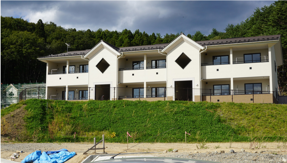
Illustration 45 | Construction of public houses in Taro District | Photo by author, October 2015
