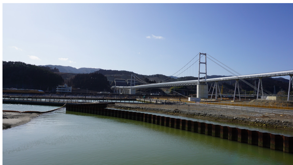
Illustration 33 | The Bridge of Hope in Rikuzentakata City | Photo by author, February 2015
