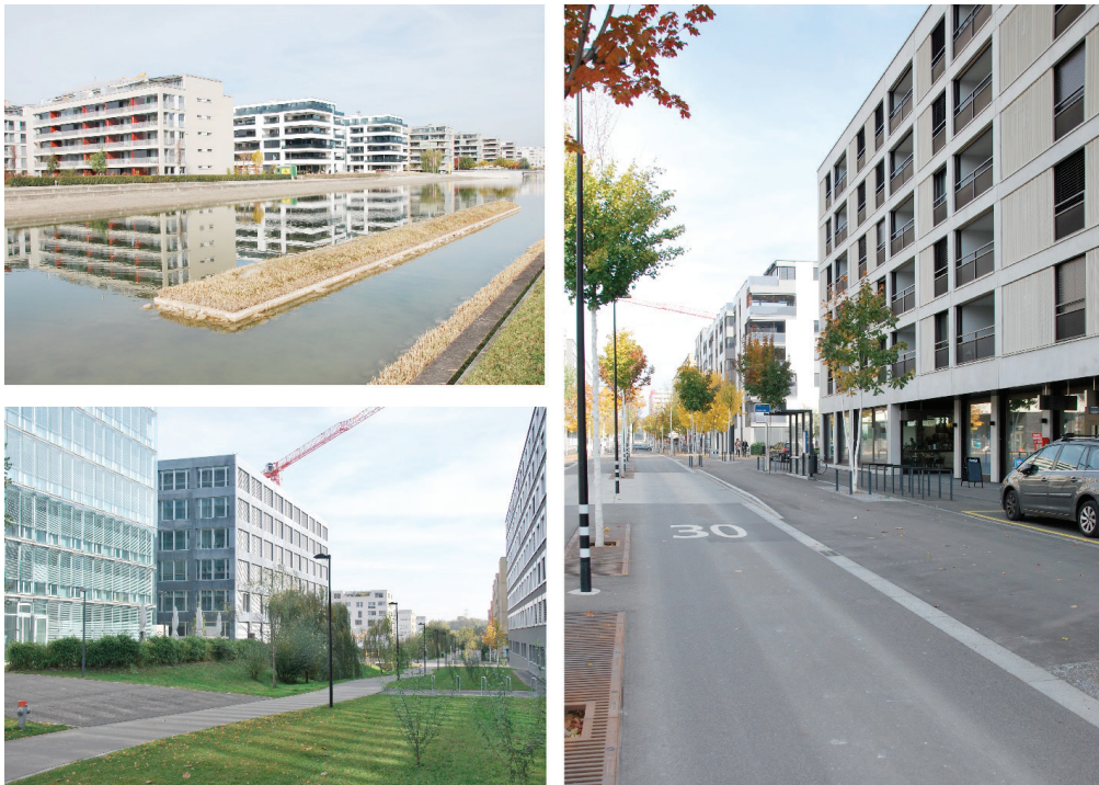
Figure 9. The three defined zones show the building design and design of public spaces in the case study of Glattpark. Source: author.
