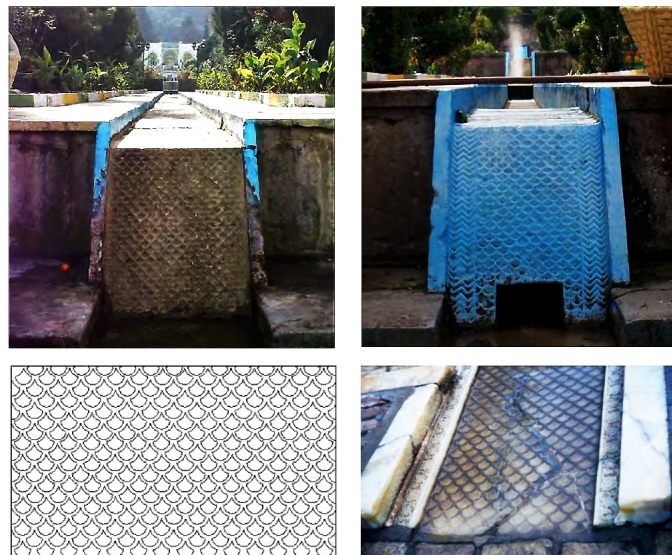
Figure 2-30 - Applying the specific featured Sequin tiles in Ashraf Garden in Behshahr (above photos) and Dolat-Abad Garden in Yazd. Embedding ceramics or rocks on the floor of streams and places where water flows for extra dynamic waves and making foams in the water (Ismailzadeh & Hosseinpour, 2016; Shahcheraghi, 2013)
