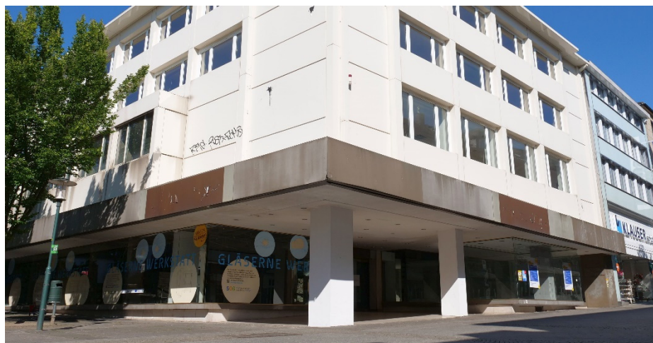
Figure 14. Former textile Department Store Solingen. Source: Stadt Solingen.
