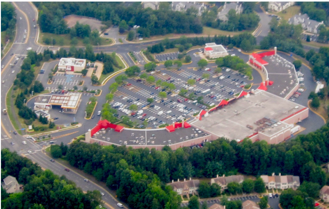
Figures 65 (top) and 66 (bottom). Post-suburbia in Clifton, VA: Notice that the different types of houses are separated from each other and that they are nostalgically themed. Neither the school (upper left) nor the shopping center (center) can be accessed other than by car. A detailed view of the shopping center (The Colonnade at Union Mills) reveals that small-town facades appear to be clued onto the otherwise completely bland facades. They have a purely decorative function and convey the dominant small town. But instead of a communal space, this row of themed facades embraces the parking lot. These photos illustrate that post-suburbia is themed to look like a small town while the different functions of a community are kept separate from each other in a suburban fashion. 2012 photos by the author.
